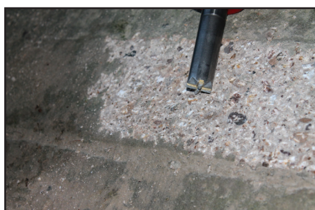
ROUGHENING CONCRETE
