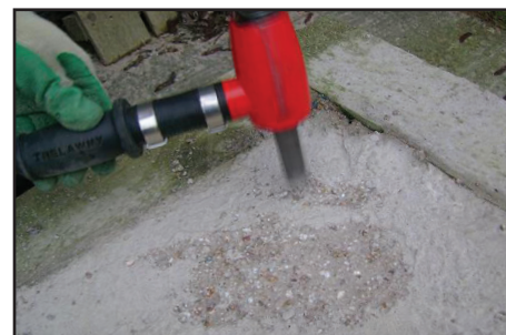
CONCRETE PREPARATION
