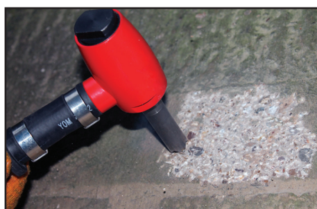
REDUCING LEVELS ON CONCRETE
